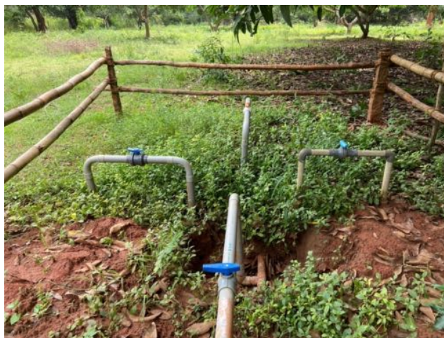
A system that connects the Mango Borewell to the existing irrigation system in the Mango Orchard and to the entire farm
